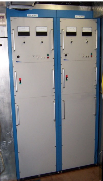
Figure 7. DTI COTS 200 kW, 20 kV power supplies.
